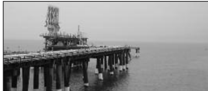
CAPITAL NEWS SERVICE PHOTO BY AMANDA SALVUCCI The Cove Point offshore pier is currently set up to receive liquefied natural gas (LNG).
