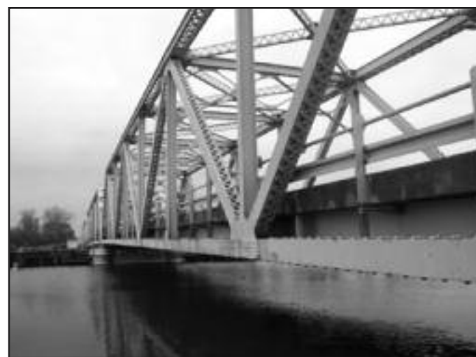
CAPITAL NEWS SERVICE PHOTO BY AMBER LARKINS. The Dover Bridge is an 80-year-old mechanical swing bridge over the Choptank River that connects Talbot and Caroline Counties.
