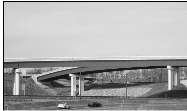
PHOTO BY DOUGTONE, FLICKR The $89 million "Contract D/E" will complete the ICC by constructing a one-mile segment between I-95 and US 1 in Prince George's County.
