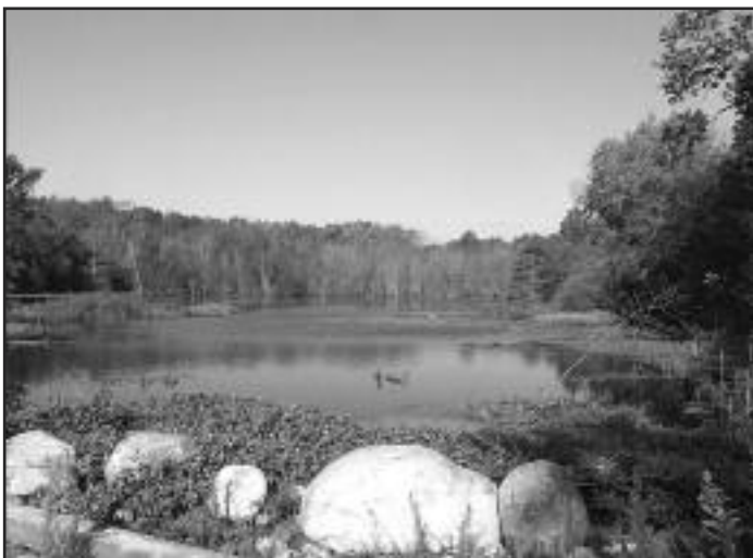
PHOTO COURTESY DEPARTMENT OF NATURAL RESOURCES Bishopville Dam Removal Project
