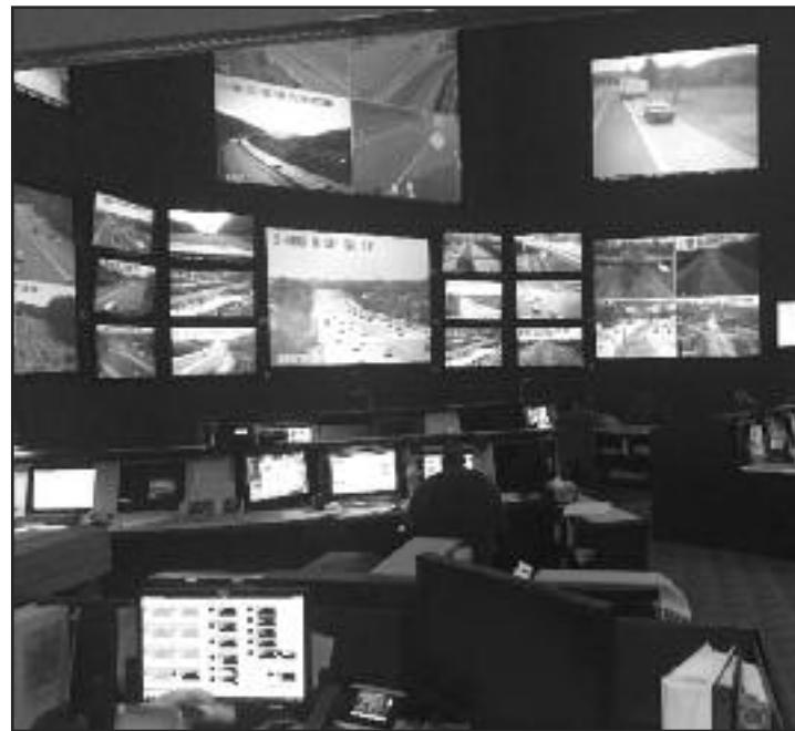
CAPITAL NEWS SERVICE PHOTO BY JOSH SCHMIDT/ The main control room for the State Highway Administration, pictured here on Nov. 8, 2017, in Hanover, Md., is where head administrators meet during winter storms to devise a plan for road cleanup
