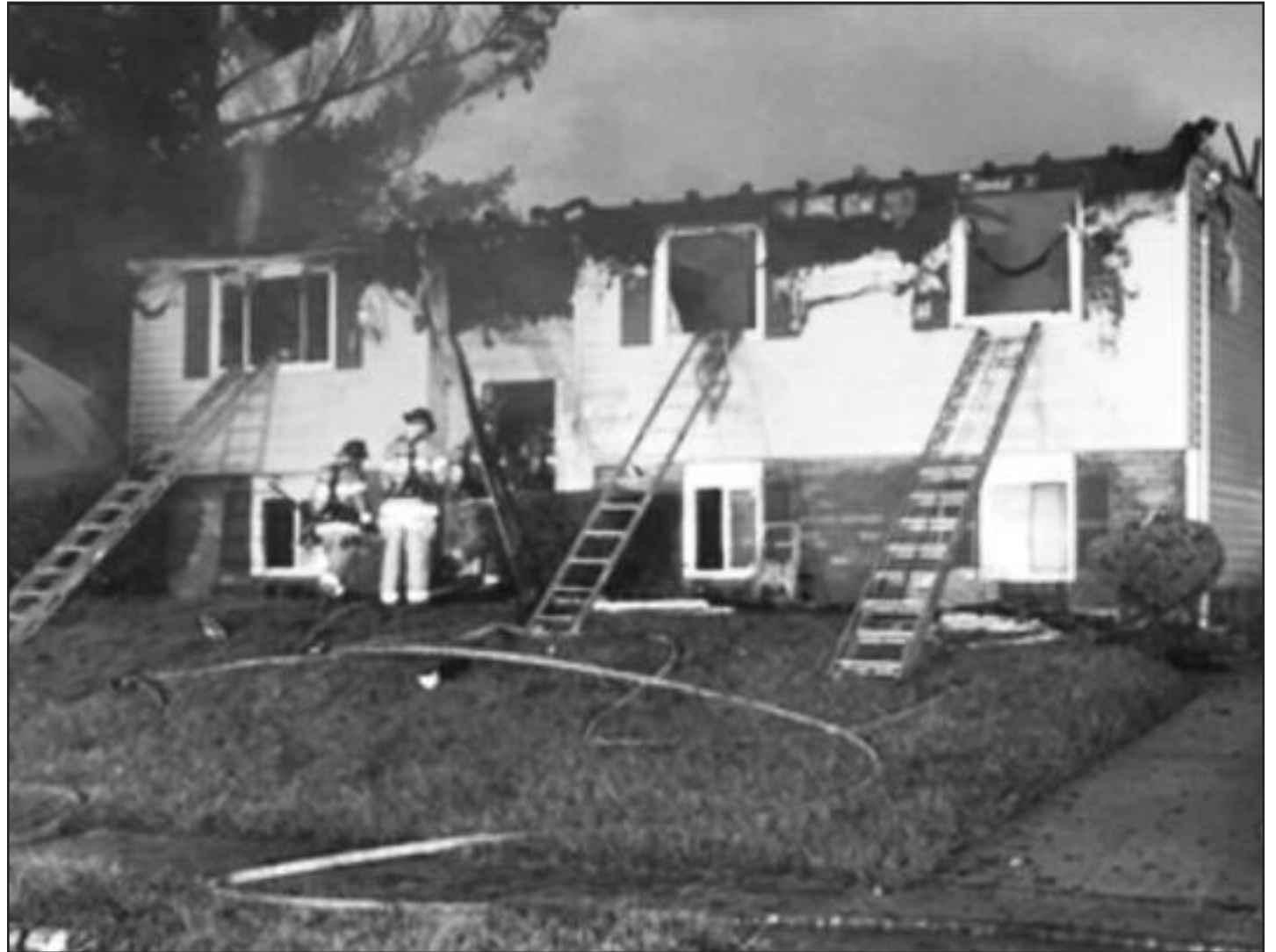
Conditions at Willow Hill Drive after fire was extinguished.
