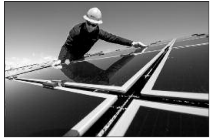
CREDIT: U.S. DEPARTMENT OF ENERGY.
