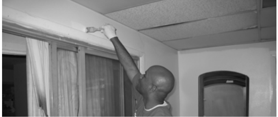
Christmas in April Volunteers Paint Kitchen. (Below) Office paints trim.
