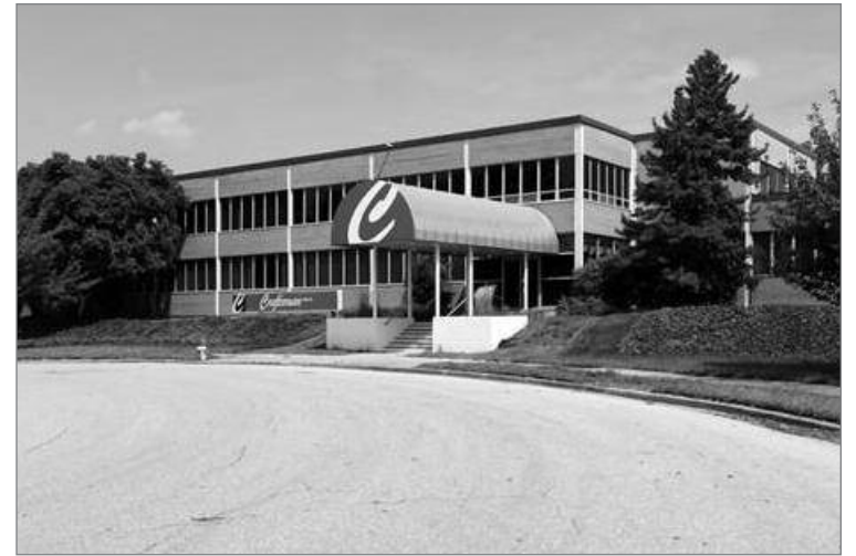
PHOTO COURTESY ATAPCO PROPERTIES, INC.
